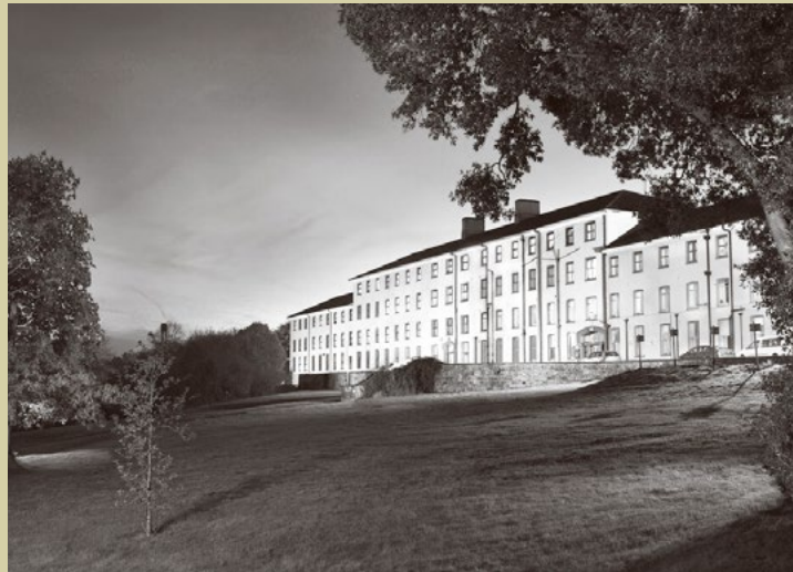
South Tipperary General Hospital
